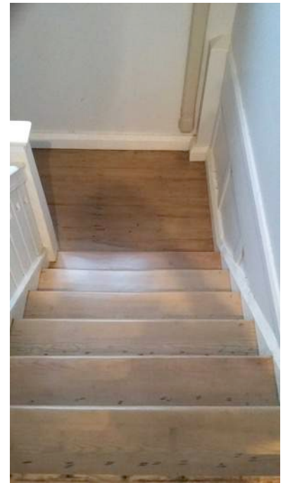
The old staircase brought back to life after sanding back and then four coats of industrial strength matt finish applied.
